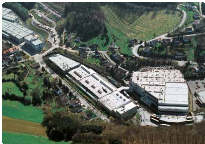
Montaplast Germany, Morsbach
