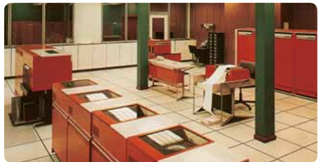
The system trend advances: In 1971, STULZ begins to specialise in the cooling of data centres. STULZ is the first supplier to introduce precision A/C systems with a flexible, modular design. This innovation puts the company years ahead of the competition.
